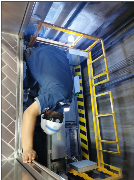
(a) Repair and maintenance work for a lift
