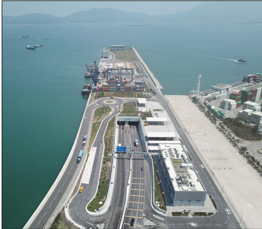
Northern landfall of TM-CLK Tunnel constructed under Contract B (April 2021)
